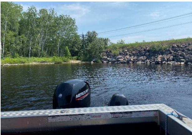
Photo 15: Looking east at the embankment on the west side of the Frog Rapids Bridge.
