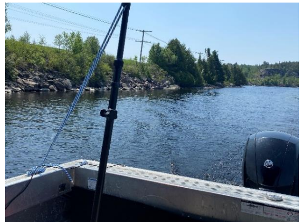
Photo 16: Looking southeast at the embankment on the west side of the Frog Rapids Bridge.
